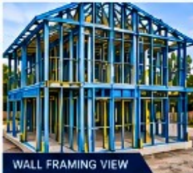
WALL FRAMING VIEW
