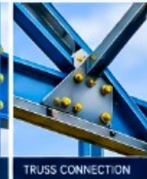
TRUSS CONNECTION
