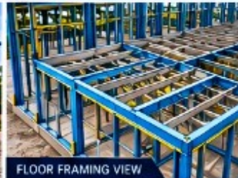
FLOOR FRAMING VIEW
