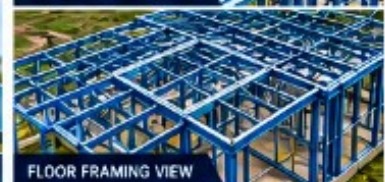
FLOOR FRAMING VIEW
